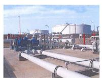
Multiphase pumps are used onshore and offshore as well as in subsea operations. Robust mechanical seals with extremely hard sliding materials have already become standard in many multiphase pumps offered by leading manufacturers. The range includes different types of single seals to buffered dual seals with pressurization via barrier fluid circulation systems.
